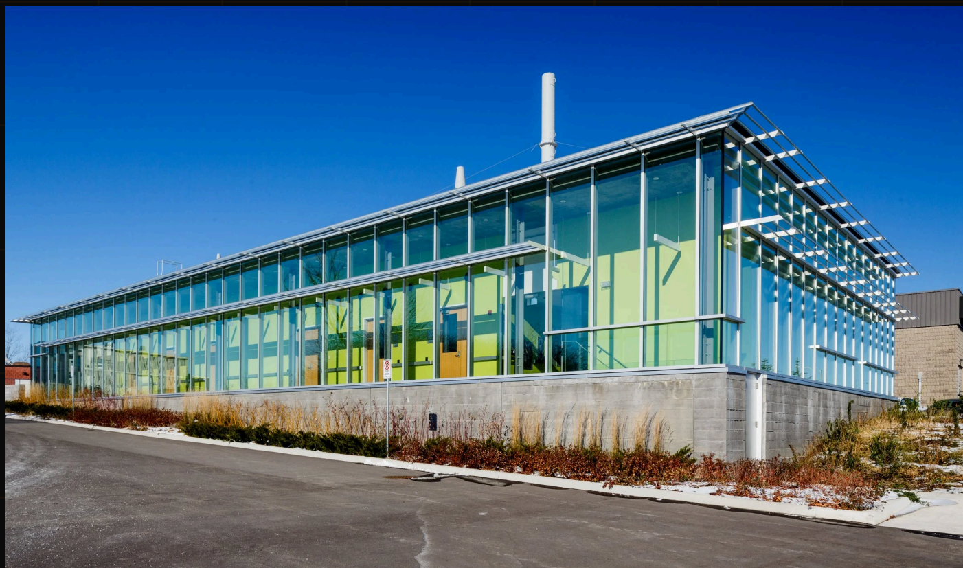
Queen's Reactor Materials Testing Laboratory located at 136 Grant Timmons Drive in Kingston, ON.
